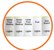
Label Circuits Clearly and Neatly for Easy Identification
